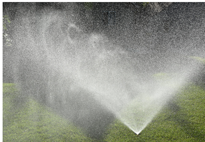
Fig. 3. Mist caused by high pressure evaporates quickly. This can result in significant water losses and is fixed by reducing pressure to manufacturer recommended levels.
